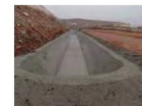
2. Salt pile La Botjosa - After the project
