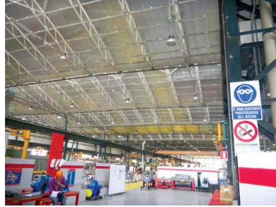
In Desio, Italy, a new roof equipped with lights is structured to increase transparency and reduce interior lighting requirements. (Interior lights are off.)
